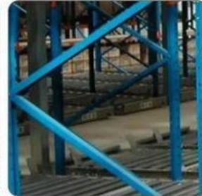
Inclined tie rod
